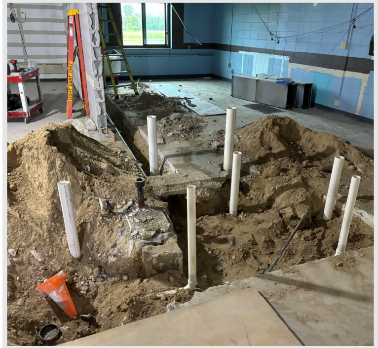
Under-slab plumbing work in one of the new restrooms.
