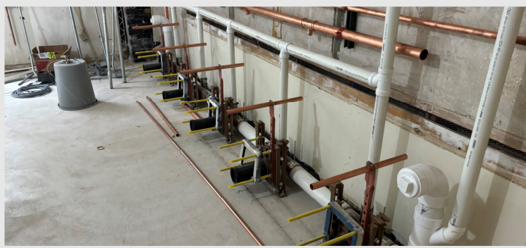
Toilet chases have been installed in what was once the Principal's Office...
