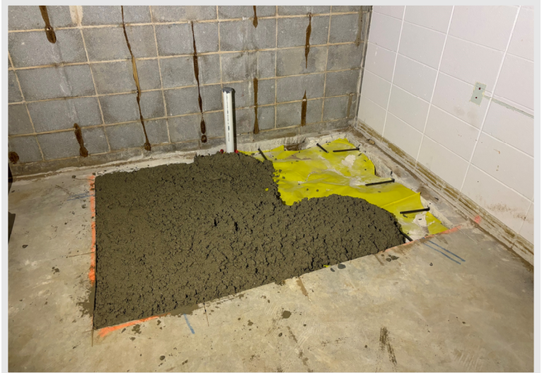
This image was caught part of the way through the slab pour-back.. It's amazing how much different that lumpy mix will change in just a few hours.
