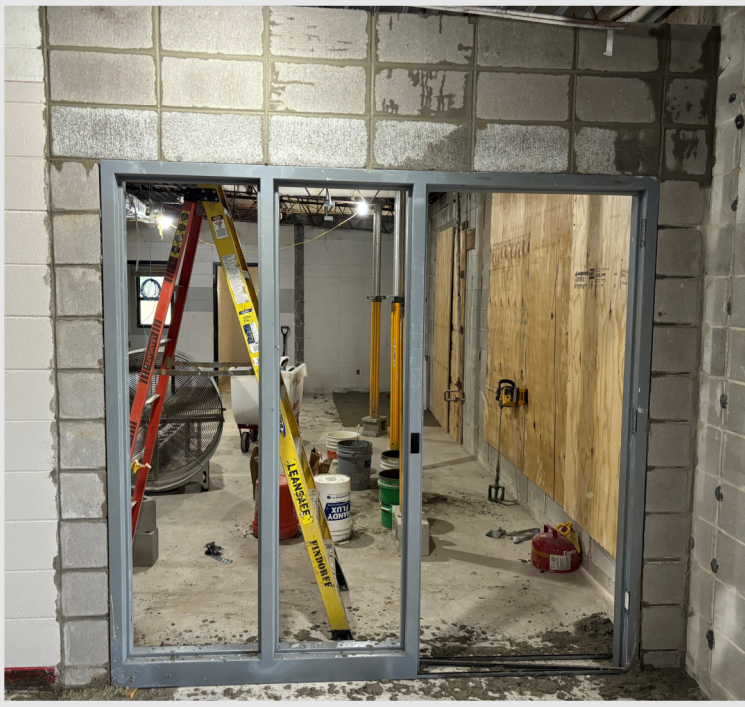
The new door in the main vestibule will allow for a secure entrance into the main office. A block masonry wall surrounds.
