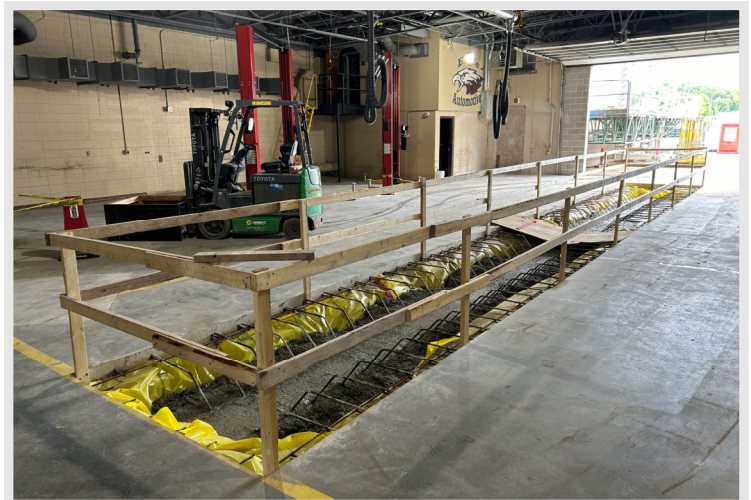
Findorff ironworker and labor crews preparing the reinforcement and vapor barrier for plumbing crews to set the new Automotive Shop trench drains.
