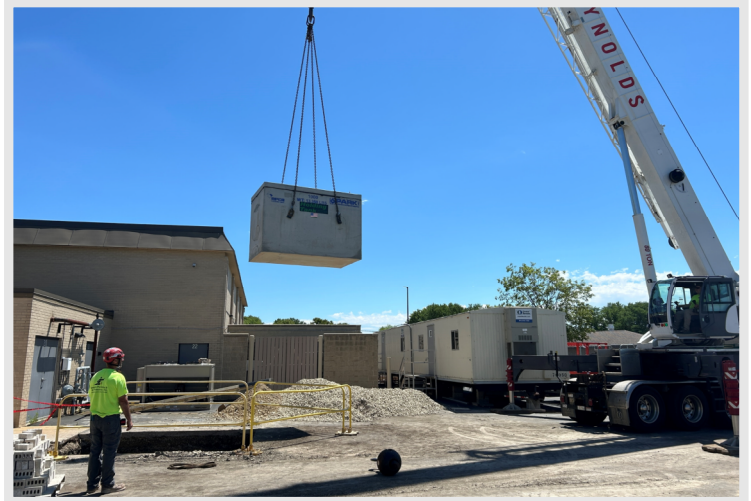
The new animal waste storage tank being hoisted into place outside of the Agriculture Shop to serve for future animal studies.
